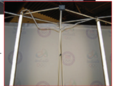
Link cable connection close up.
